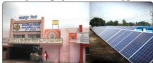
25 KwP SPV Power Plant at Railway Station under PSU CSR
